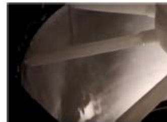
Properly adjusted TXV
