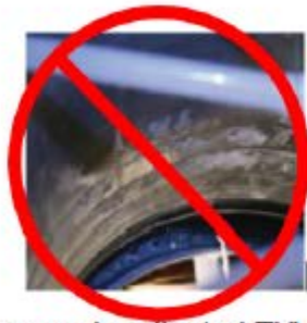
Improperly adjusted TXV
