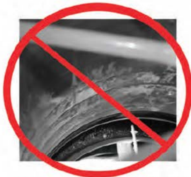
Improperly adjusted TXV
