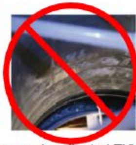
Improperly adjusted TXV
